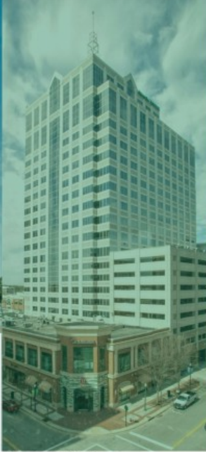
Armada Hoffer Tower
